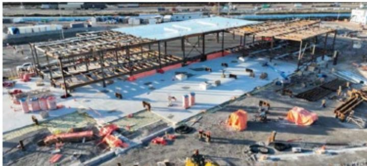
At the hospital, steel for the main structure has advanced. The team is also protecting the work from frost with insulated tarps.
