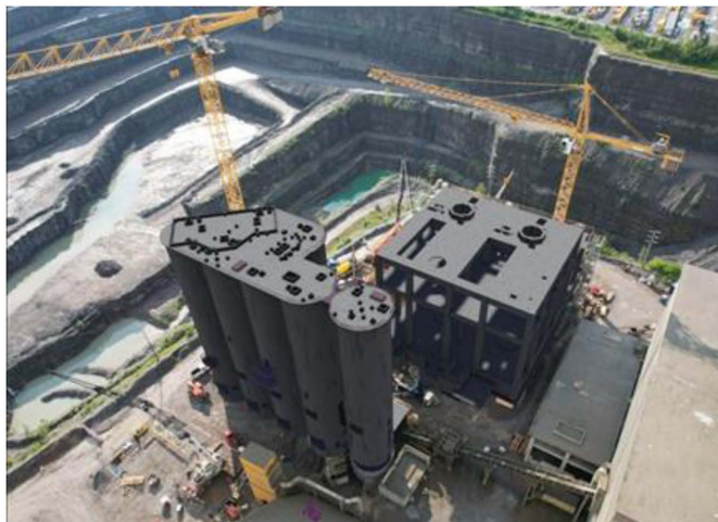
Fig. 2. Concrete silo structural BIM model view superimposed on a drone aerial photo. (Images by authors.)
